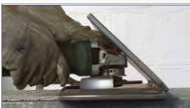
Typical problem...Grinder doesn't reach
